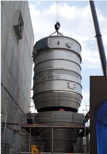
Spray Drying Tower Assembly (Lübbbers)
